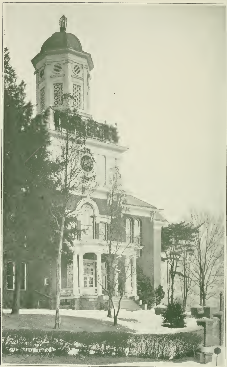
CARVER HALL—ERECTED IN 1867
