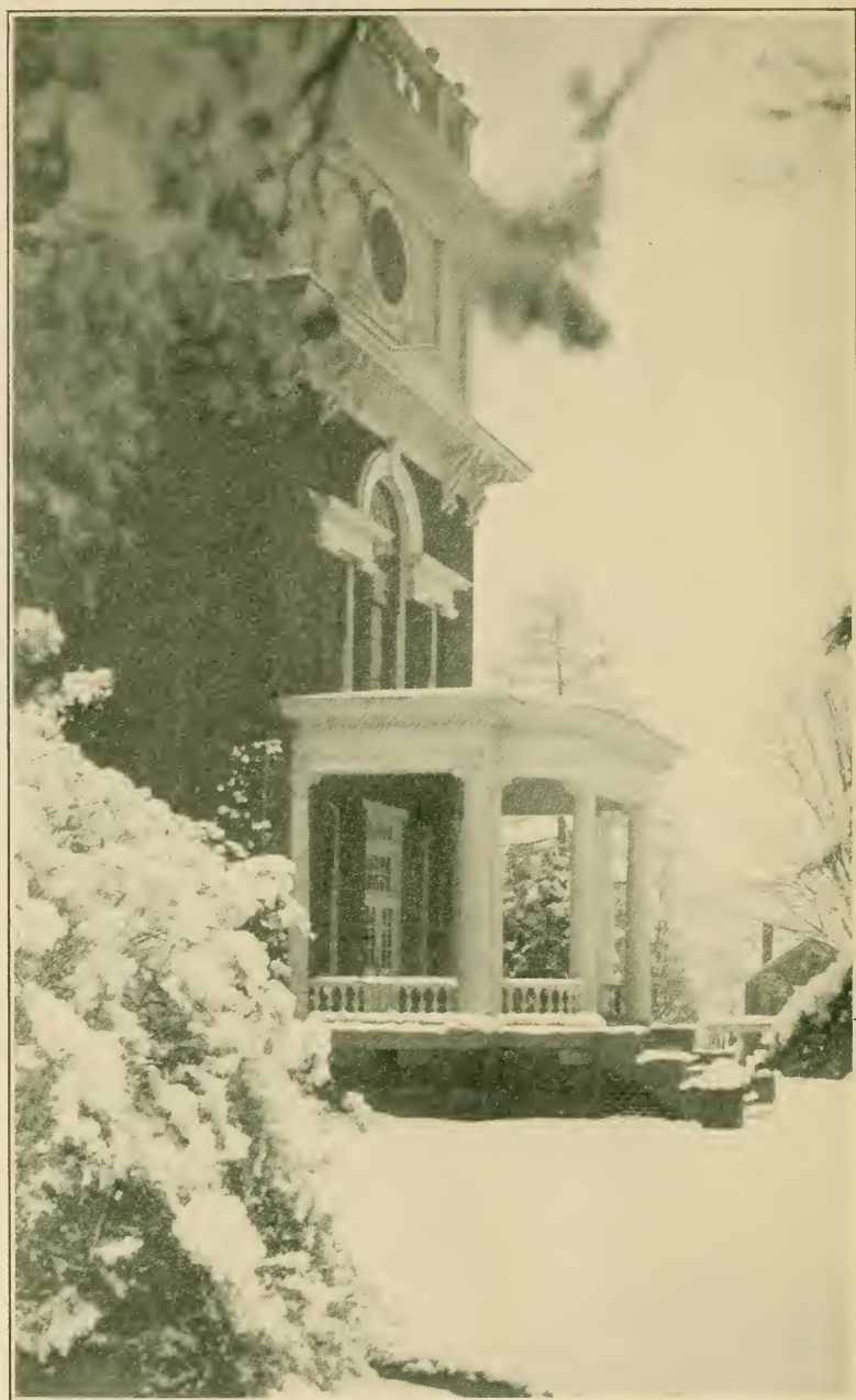
CARVER HALL—ERECTED IN 1867
