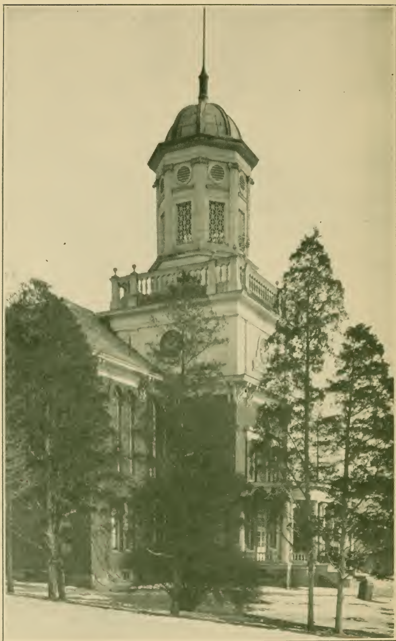
CARVER HALL, ERECTED IN 1867
