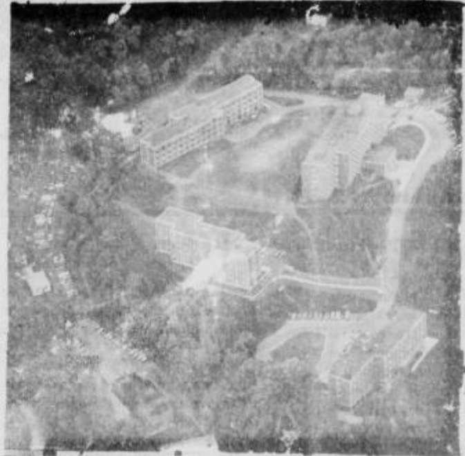
EAGLE TAKES TO THE AIR: A fly over the campus gives people a different perspective of "the hill" which shows Lock Haven's newer housing facilities. This flying photo was made possible by pilot Lynne O'Donnell, a Piper secretary. Photo by MARC MUSHENO.
