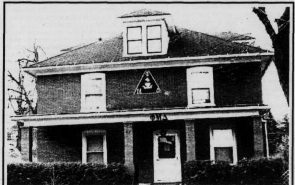
Fraternities, such as Phi Mu Delta, are currently being given "courtesy inspections" as a predecessor to the new rental inspection ordinance (photo by Karl McCollester).
