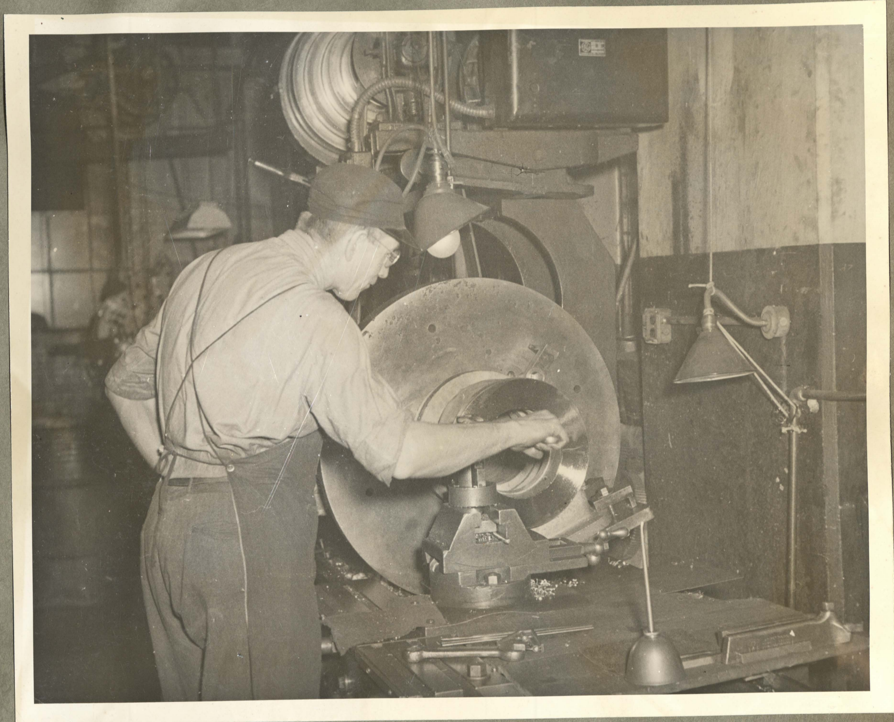
MACHINING 6" VALVE CASE
