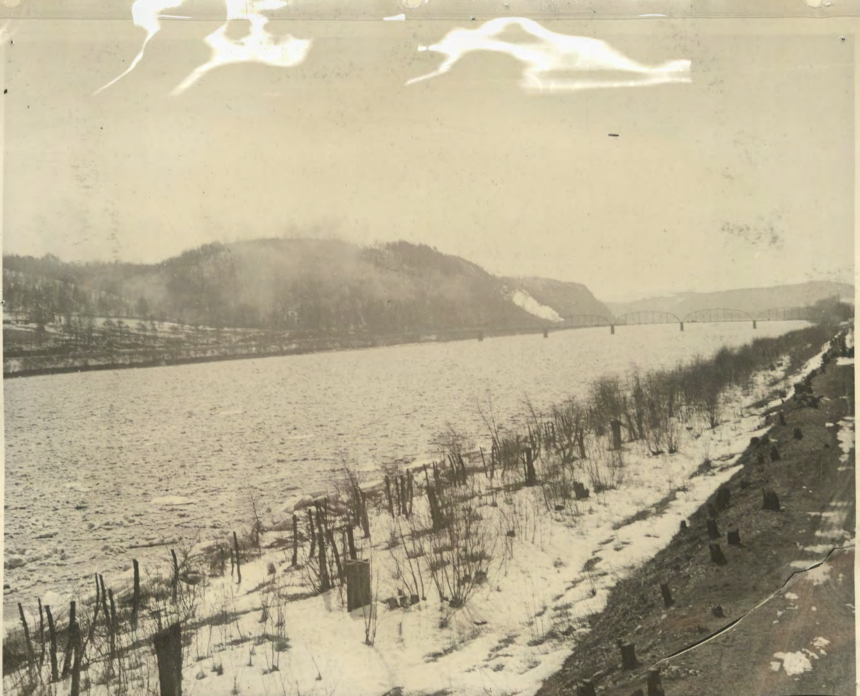
FLOOD IN FIRST STAGE
