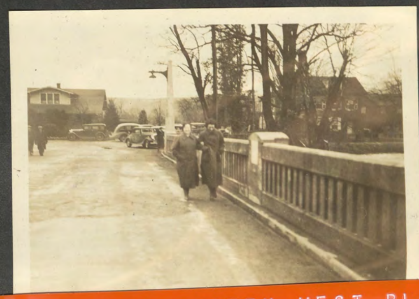
BRIDGE - CREEK WEST BLOOM
