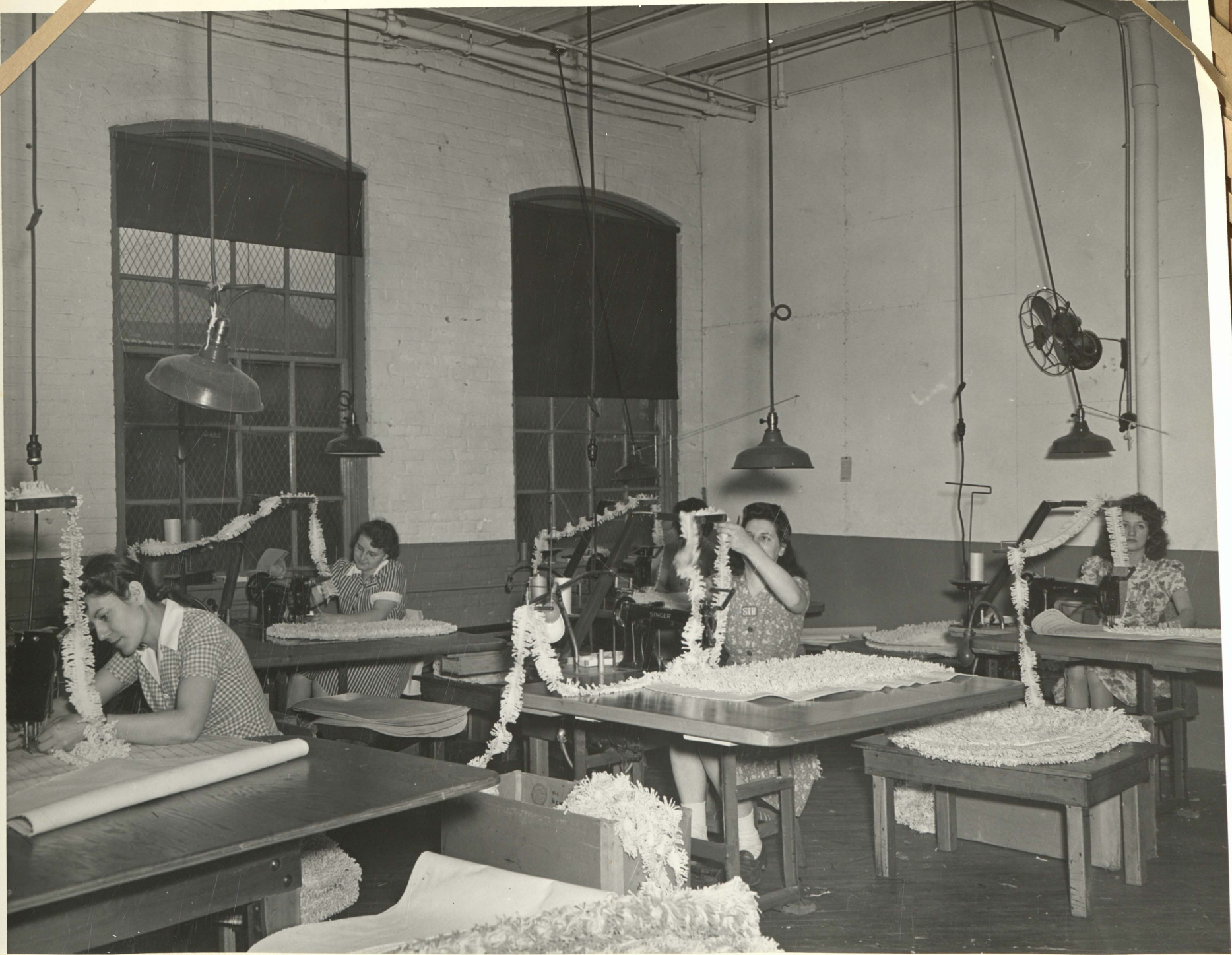
View of a section of the cotton rug department showing operators sewing fringe on duck backs.
