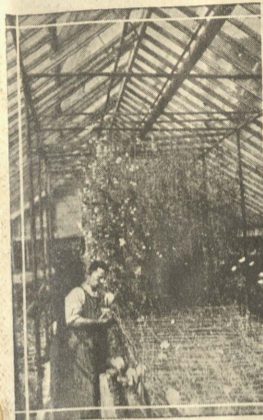
Interior view of the greenhouse.
